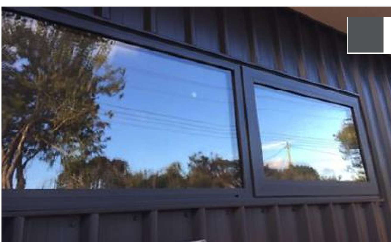
09 POWDERCOATED ALUMINIUM FRAMED DOORS/WINDOWS - BASALT
